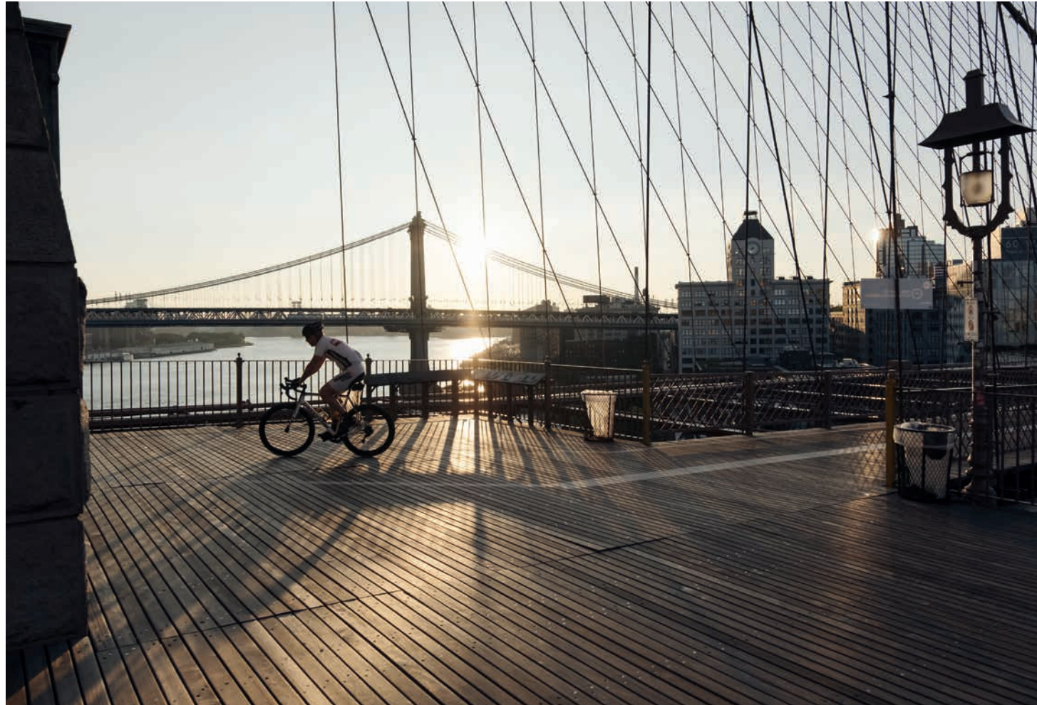
The Brooklyn Bridge forms a key link between the boroughs. Along with 100,000 or so cars, more than 4000 pedestrians and 2600 cyclists make use of the bridge every single day, via an old-fashioned boardwalk made of more than 11,000 hardwood planks, which are replaced every 35 years.
